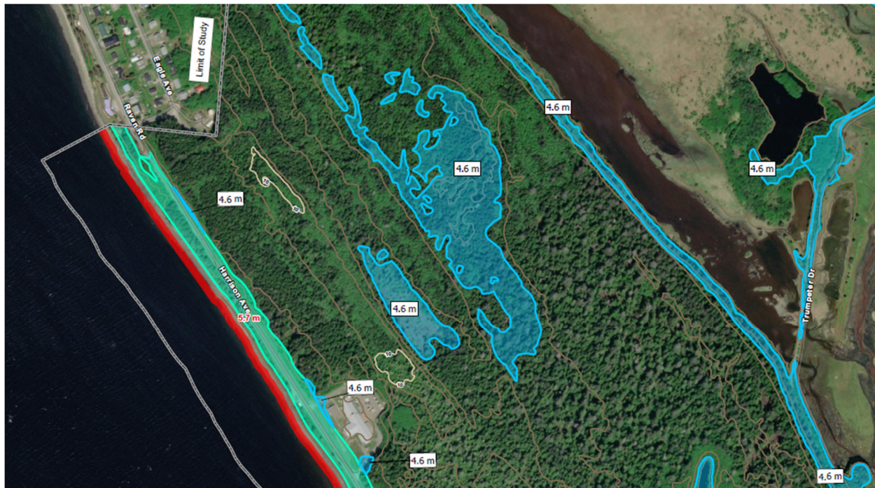
Figure 2.4 Portion of map showing the coastal FCL with 1 m of SLR at the northern segment of shoreline fronting Masset Sound. These results show that the Masset Medical Clinic is not within the FCL zone but that Raven Road, which provides access to the clinic from Masset and Old Massett would be impacted.
