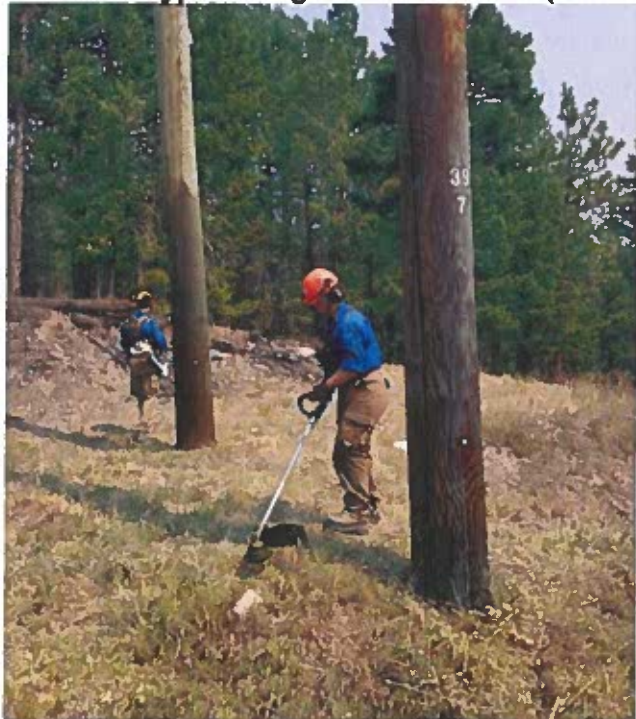
Photo 1: Typical vegetation removal (brushing)
