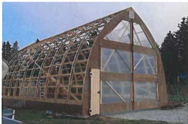
Fig 1.4 example of a bow-roof shed frame. This one is considerably taller than the one proposed.
