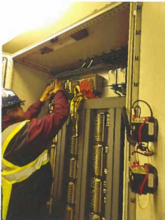
Wiring in the new PLC
