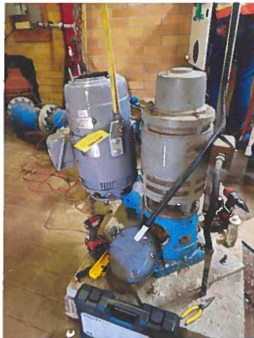
replacing 480V distribution pump with 600V pump
