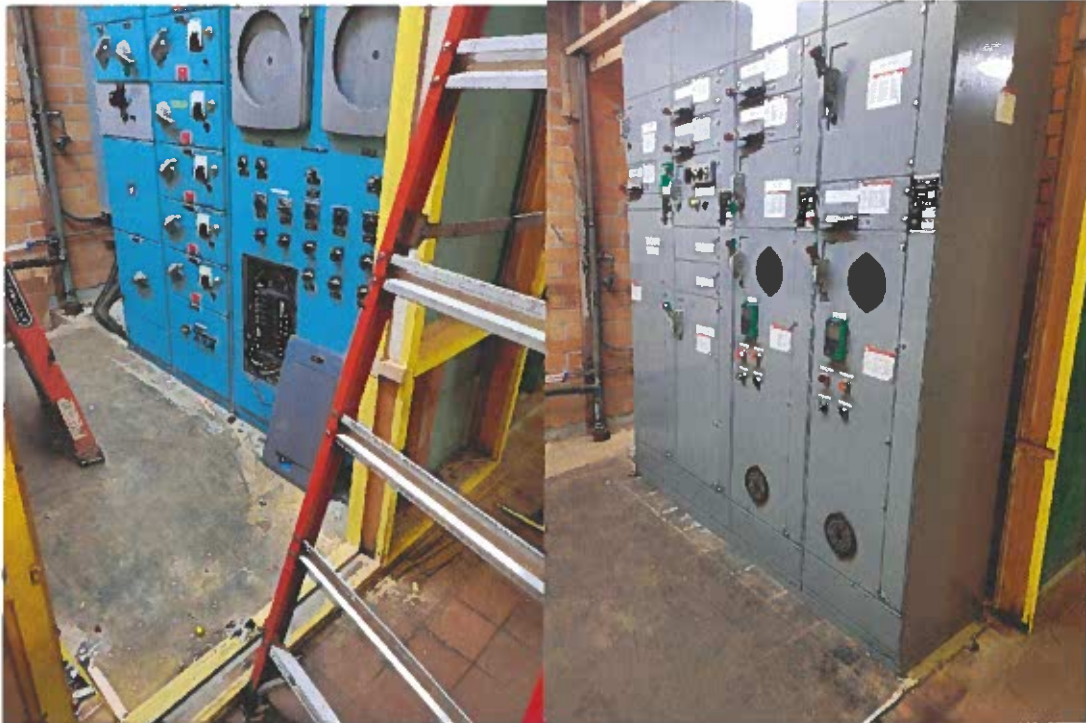
Replacing old 480Volt – 3Phase MCC (left) with 600Volt – 3Phase MCC (right)
