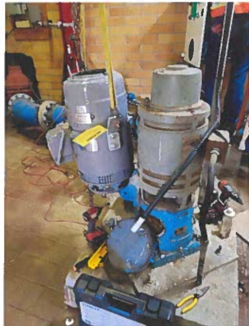
replacing 480V distribution pump with 600V pump
