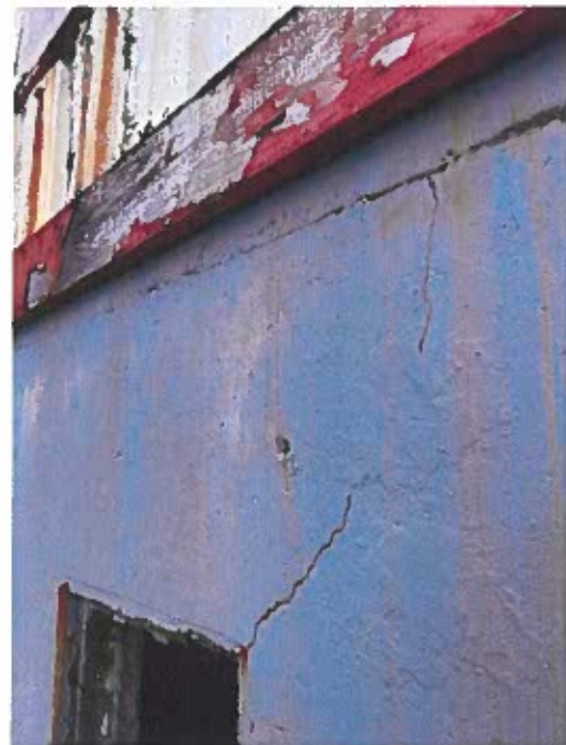
Figure 4: Foundation Cracks
